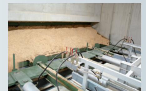
Hydraulic discharge activator (push-floor system)
