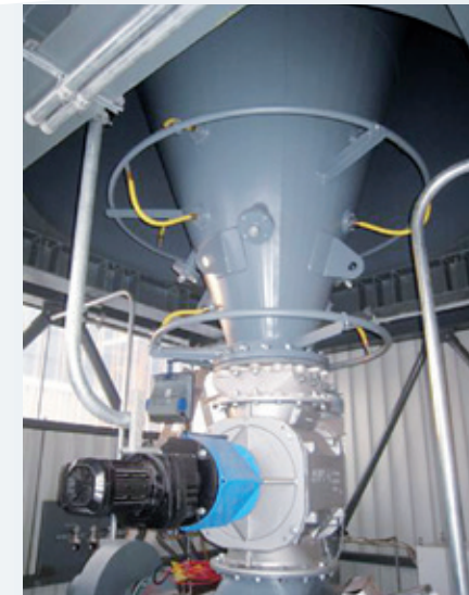
Silo discharge with gate slides and rotary valve
