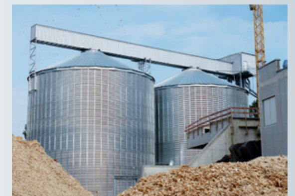
Pellet storage and loading silo works with filling and loading technology
