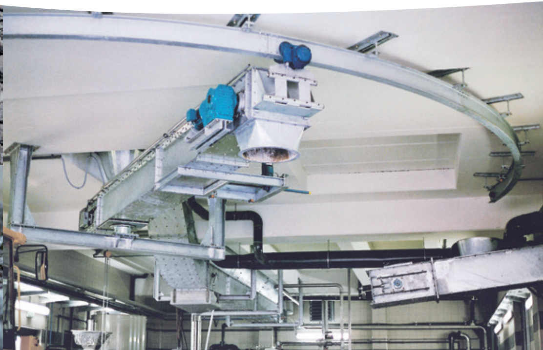
Loading station for sewage sludge with articulated chain conveyor in a sewage plant
