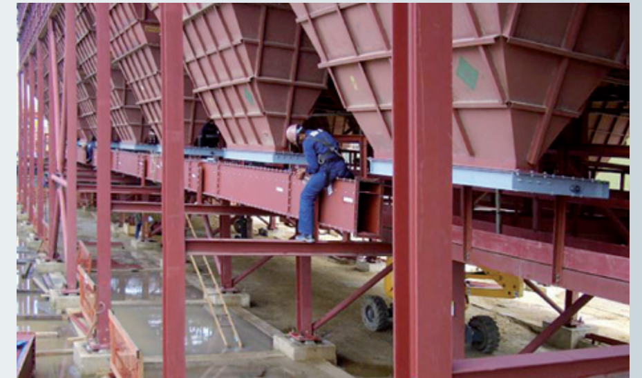
Installation of a chain conveyor in a filtration system
